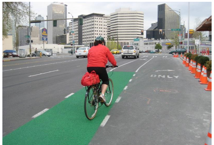
Bike lanes should continue all the way to intersections (above) and should be dashed where they cross right turn lanes. Green pavement (below) can also be used to highlight conflict areas.
