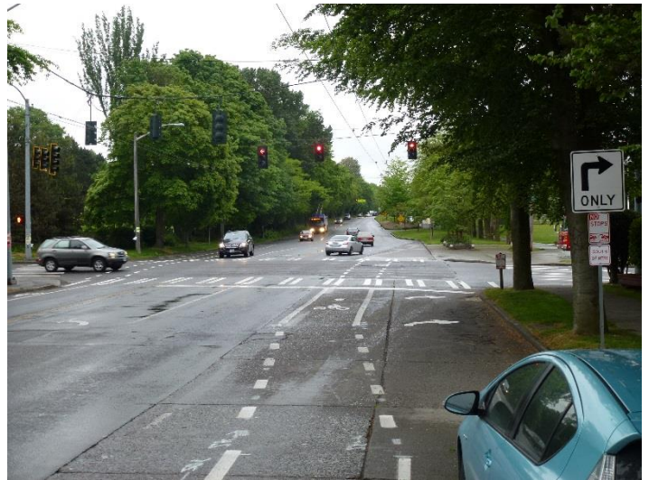
Bike lanes should continue all the way to intersections (above) and should be dashed where they cross right turn lanes. Green pavement (below) can also be used to highlight conflict areas.
