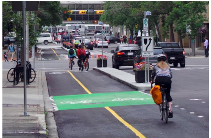
Separated bike lanes are typically used on large multi-lane arterials with high vehicle speeds, but can be appropriate for lower-speed streets that have high traffic volumes.
